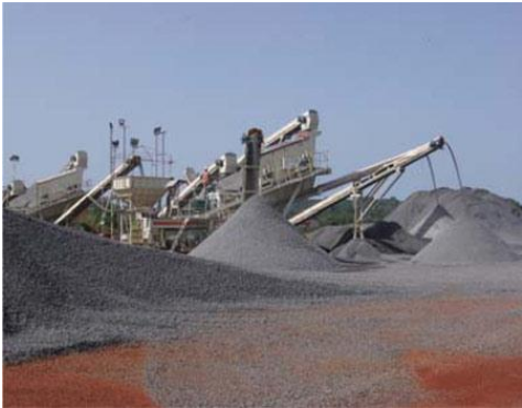
Earthworks crusher operations from http://www.globalalumina.com/gallery.php
