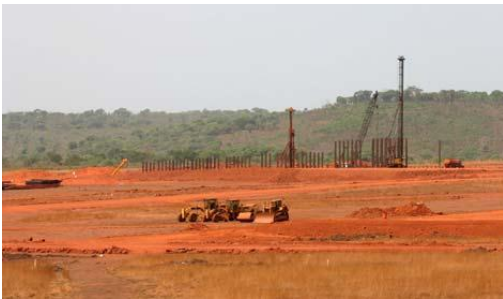
Overview of refinery areas and piles from http://www.globalalumina.com/gallery.php
