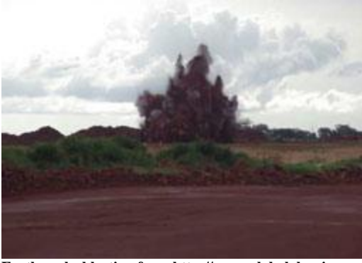
Earthworks blasting from http://www.globalalumina.com/gallery.php
