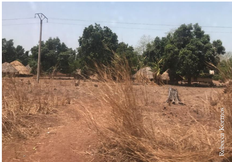
Hydroelectric power lines in Guinea run above houses, providing electricity for only 3% of Guinea's rural population.
